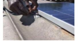
3. Connect the cables from the solar panel and incubator to the control unit.
